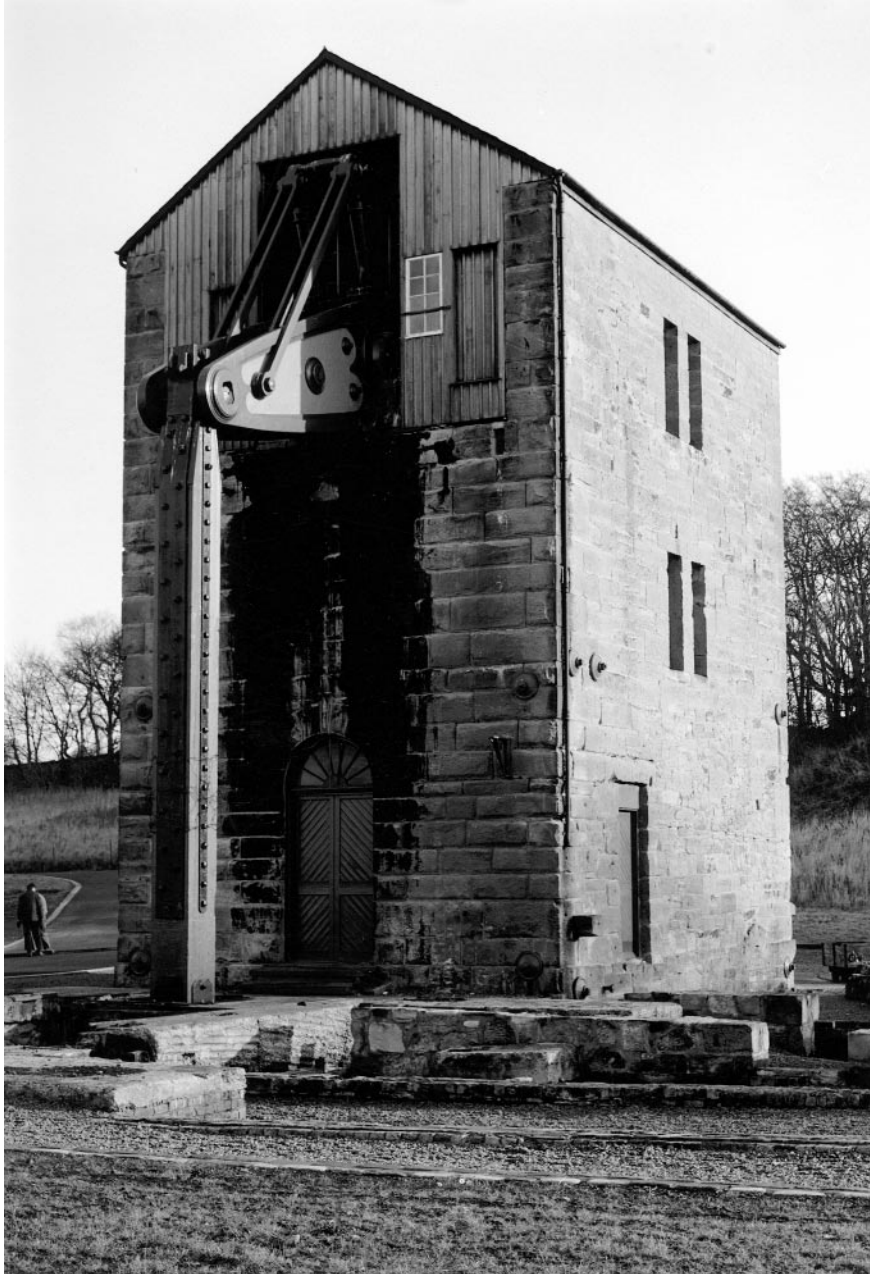
Beam Engine exterior East Lothian Council
