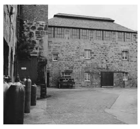
The Fowler's Brewhouse on the north side of the main street in Prestonpans. The louvred windows allowed the air to cool the malt liquor before fermentation
