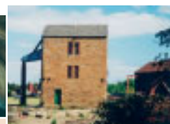
Prestoungrange beam engine
