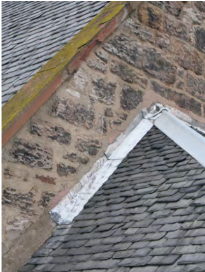
Detail of abutment to roof at N gable
