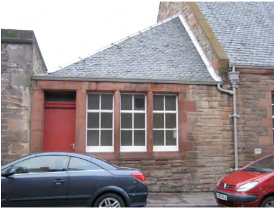
East elevation of kitchen
