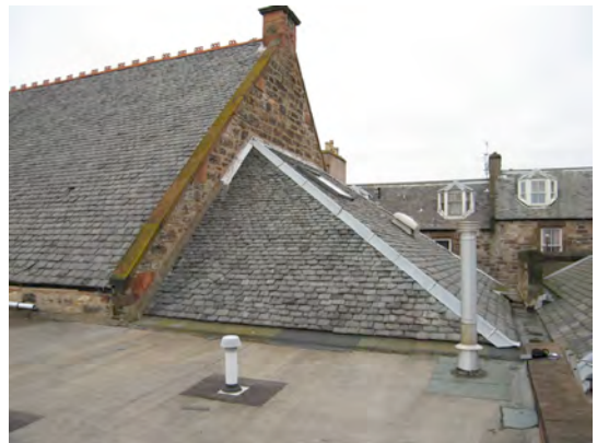
View of roofs looking WNW
