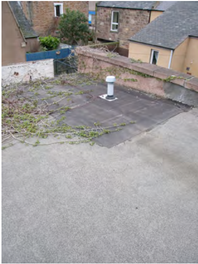
Landing roof looking NW showing felt patch to mastic and vegetation
