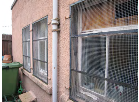
Windows to caretaker's store and ladies toilet on S elevation
