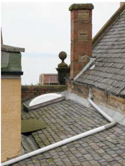
Detail of N lobby roof showing rooflight
