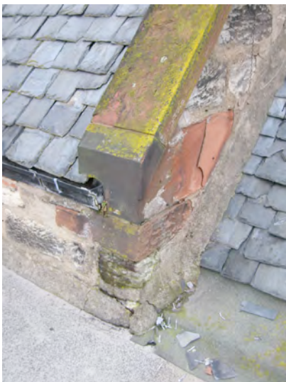
Detail of SW skew and gable showing poor fillets and flashings and masonry decay
