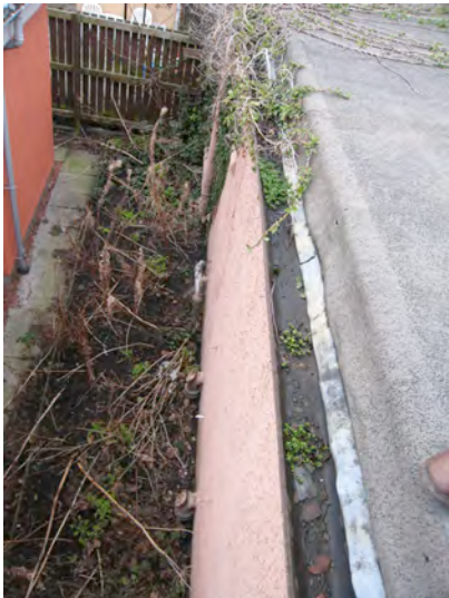
West low level eaves showing blocked rhone and vegetation
