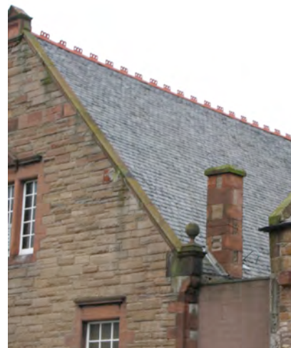
Detail of NW skew and chimney
