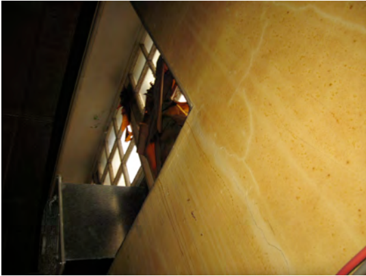
Detail of hall high level N window
