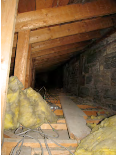
Roof space over bar showing blocked windows
