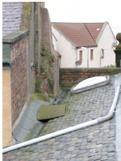
Detail of abutment to NW showing rooflight, rainwater pipe and felt weatherings and gutter at abutment
