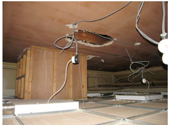
Ceiling void over ante room showing damage to upper ceiling
