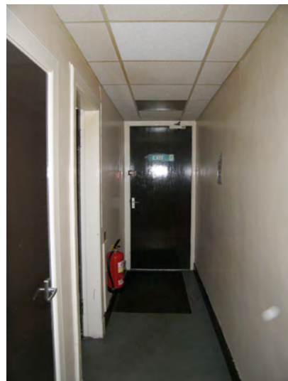
Rear lobby looking E
