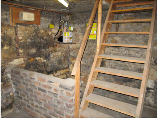
Basement looking NE, showing stair and gas meter
