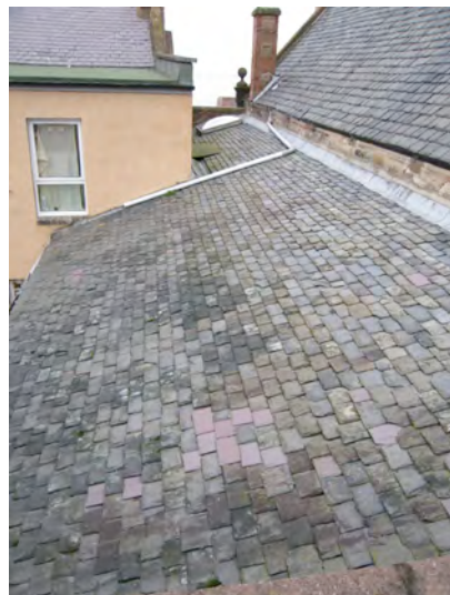
Bar area roof looking W
