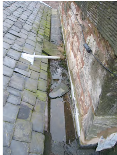
Detail of S roof felt gutter
