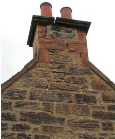
Detail of chimney showing movement to chimney and cope
