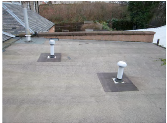
Landing roof looking S, showing ventilation terminals and flue
