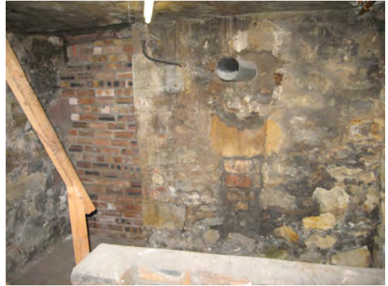
Basement looking SW, showing blocked door and open flue
