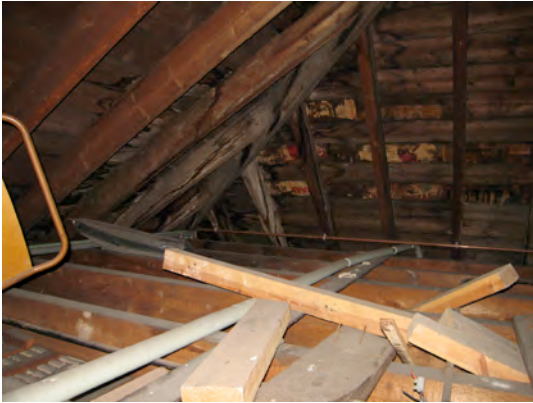
Roof space over ante room
