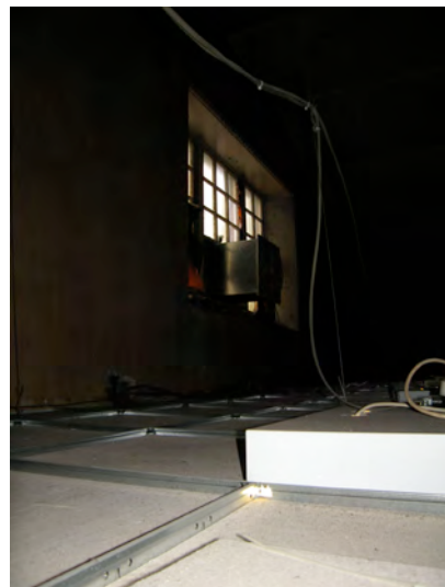
Hall high level N window
