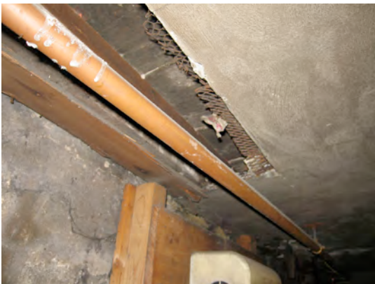
Damaged plaster to basement ceiling
