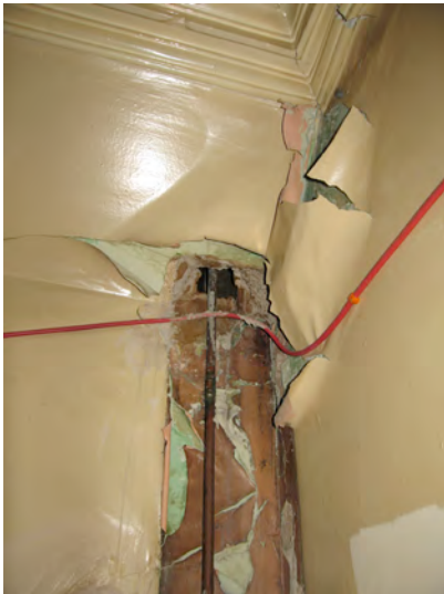
Ceiling void over ante room showing typical damage at services
