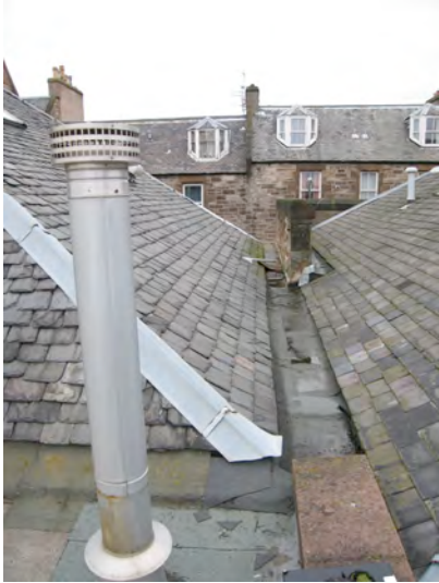
Felt valley gutter to S and boiler flue
