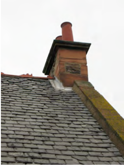
Detail of N gable chimney
