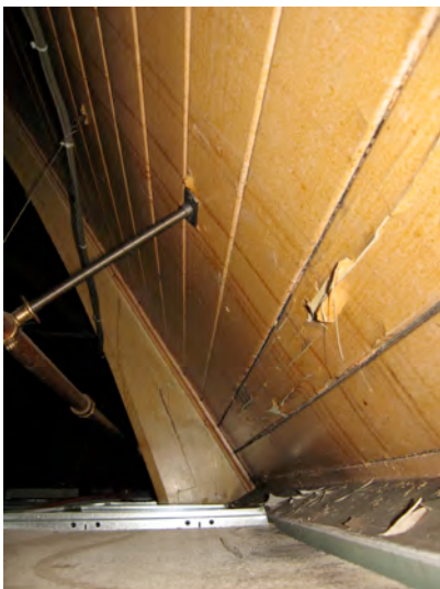
Detail of hall upper ceiling and roof truss
