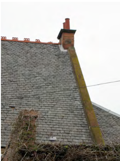
Detail of SW skew, ridge and S chimney
