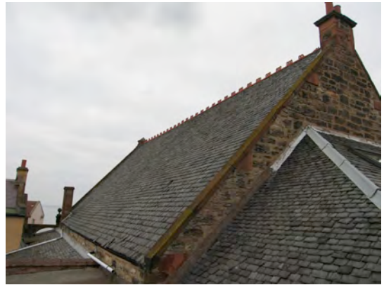
View of roofs looking NE
