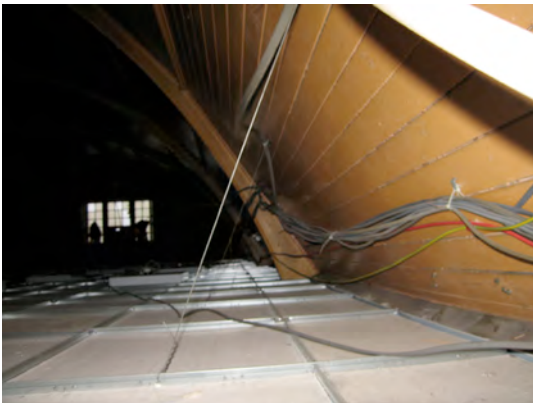
Ceiling void over hall looking N
