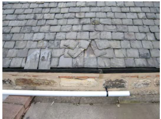
Detail W pitch eaves showing slate work, masonry decay, rhone and plastic rainwater pipe
