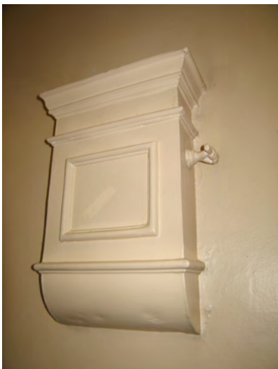
Detail of ventilators to hall
