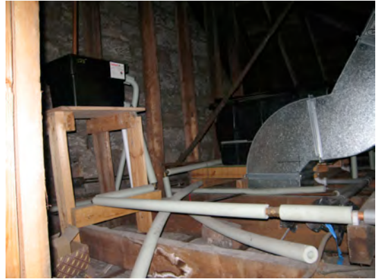
Roof space over kitchen showing extract
