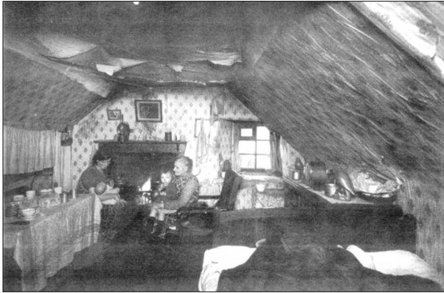
Example of the effects of neglect and lack of maintenance in early Miners' Housing
