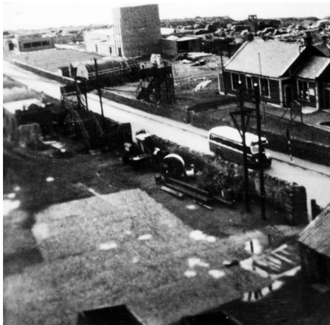
View of Prestongrange featuring NCB 'improvements' such as (from right) Road Transport, Bathhouse, Cafeteria
