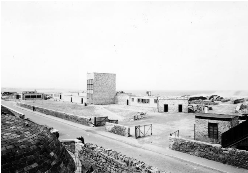
Pithead Baths, Canteen and Pipe Store on the shores of the Firth of Forth Scottish Mining Museum Trust
